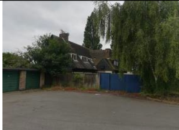
Rear of public house from garage block site
