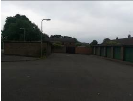
Garage block site looking north
